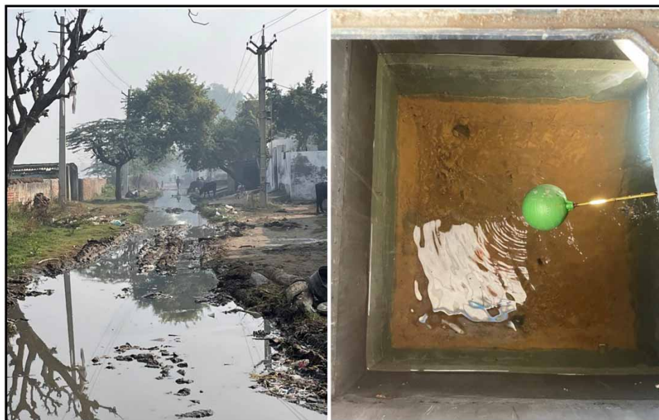
Figure 8 | Photographs of cattle and the flooded access road in front of the school in Kiranki (left) and the interior of the tank at Saramthala that contains biofilm, sludge, and often has mosquitoes and other insects (right).
