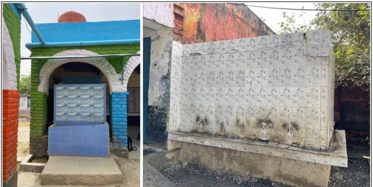
Figure 2 | Examples of rainwater (left) and groundwater (right) supplied drinking water tanks at schools in the study area.
